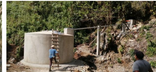
New tank which we have already built to collect water from the spring
